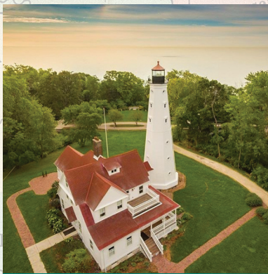
North Point Lighthouse
