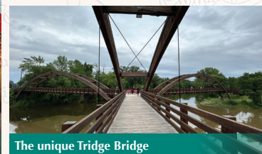
The unique Tridge Bridge
